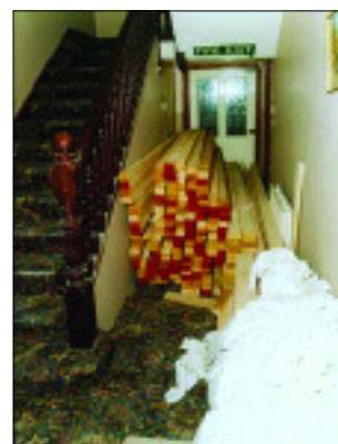
Figure 9: A blocked corridor with incorrect signage
